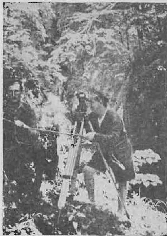
Fig. 6. Ridicînd profile transversale
