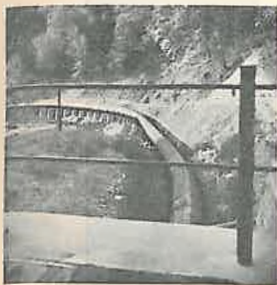
Fig. No. 4. — Conducta pleacă dela baraj.
