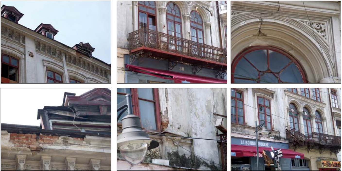
Fig. 20, 21, 22, 23, 24, 25, 26 - Tipuri de fracturi, unele extrem de periculoase
