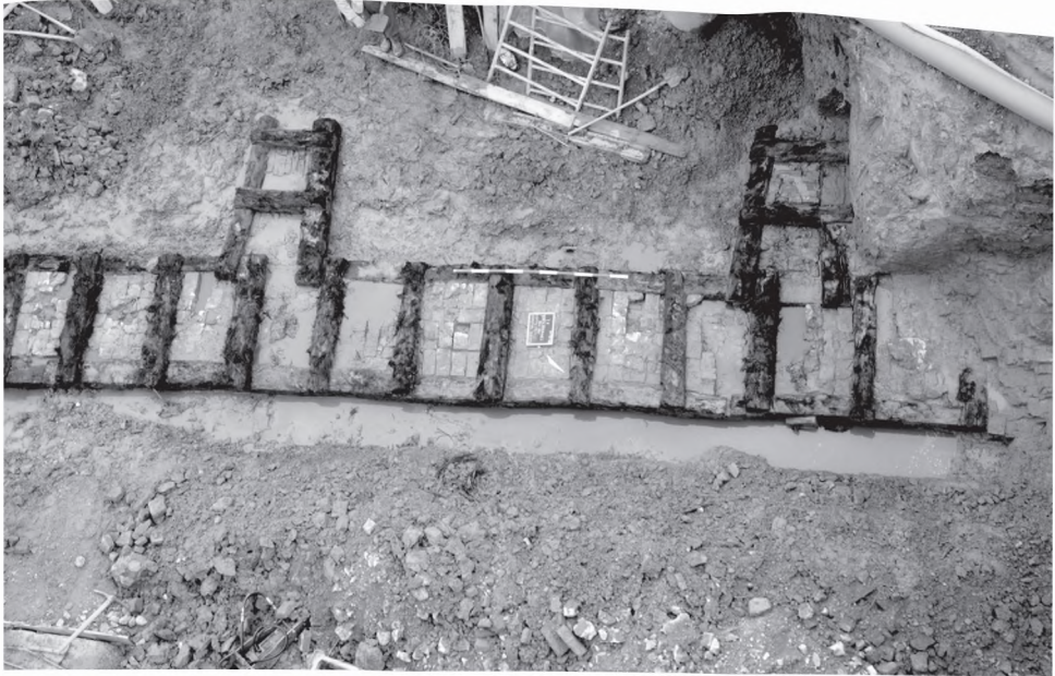
Pl. VI. 1. Lonjeroanele substructurii de lemn a contraescarpei; 2. Contraforturile de la contraescarpa contragardei I. / 1. The longitudinal beams of the counterscarp wooden substructure; 2. The counterforts of the counterscarp of counterguard I.
